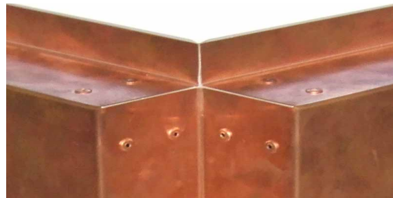
Examples for the rivet arrangement as a function of the corner cut for peripheral bent edge formats
