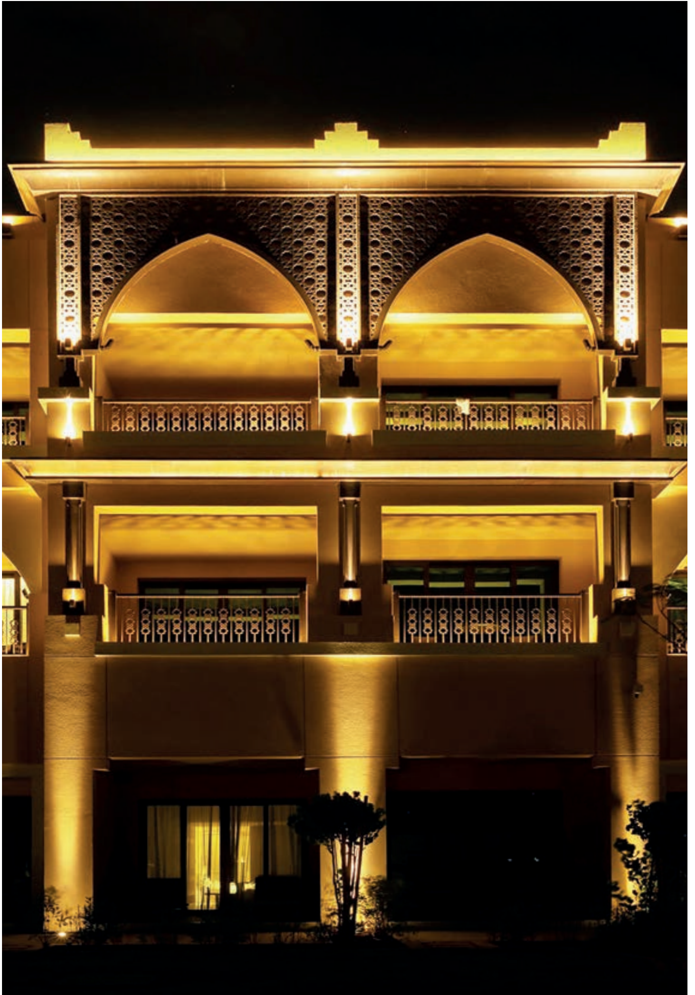
Uplights and in-ground lamps
