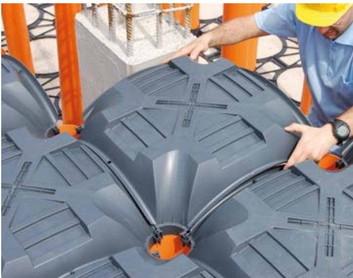
The formwork and bases can be cut/shaped according to the design characteristics. The modifications shall be made as specified by Geoplast (see Appendix C) using an angle grinder or disc cutter.
